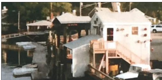
(Upper) Harbormaster's Office under construction (Lower) Completed building with bird houses
