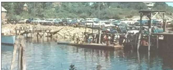
Swing boom hoist added in the mid-1950s
