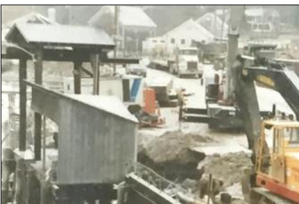
Work begins on new bait cooler, roadway and bulkhead
