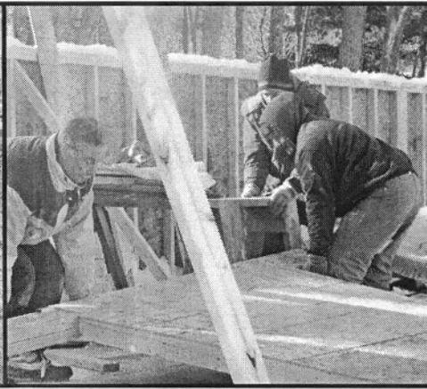
The front wall raised one cold winter day...
