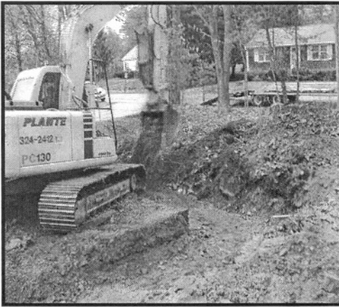
The excavation the day before Thanksgiving, 2004...
